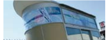
Can be installed in a day
